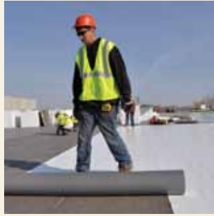
2. Apply membrane, overlapping seams in the direction of water run-off.
