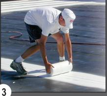
inforce seams with Spunflex<sup>®</sup> embedded in Rapid Roof® III Base Coat or Equinox<sup>®</sup> Base Coat.
