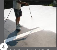
Seal entire roof with Rapid Roof® III Top Coat or Equinox<sup>®</sup> Top Coat
